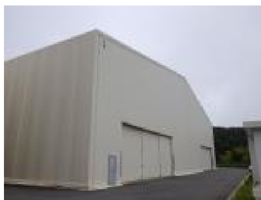
No.2 陣場沢仮設灰保管施設a①
